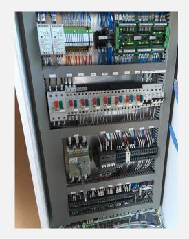
All electrical equipment reliably performs its work to provide plant power supply and microprocessor control of power units. The set of electrical equipment of the plant includes more than 350 items of purchased units. As the development of our plant, the schemes are constantly improving.
